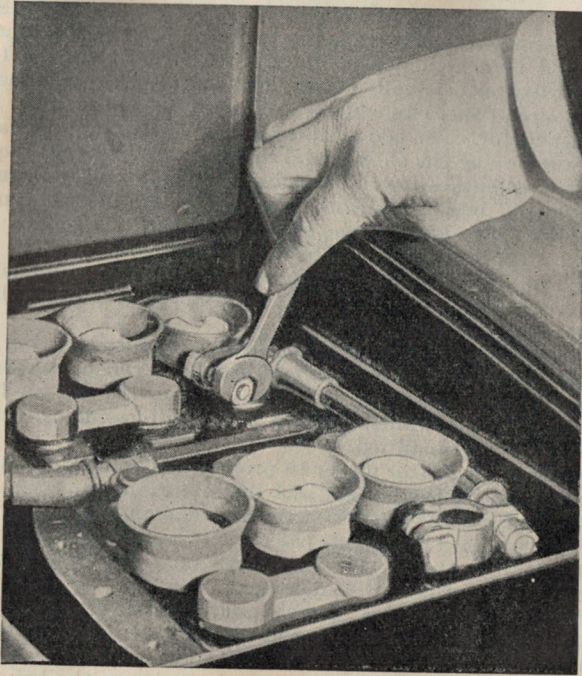
FIG. 76. TIGHTENING A BATTERY CABLE CONNEXION
